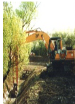
Land Drainage Works
